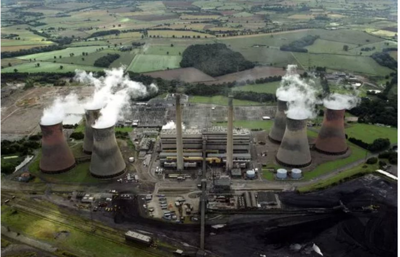
Plate 2: Aerial Photo of Drakelow Power Station C – Looking south to Site
